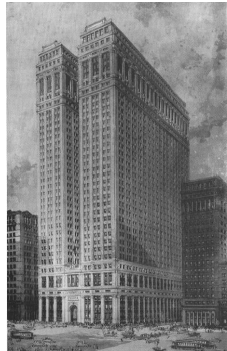
Figure 1: Equitable Life Assurance Building. New York, completed 1915, architect Peirce Anderson of Graham, Burnham and Co. Photo: New-York Historical Society
